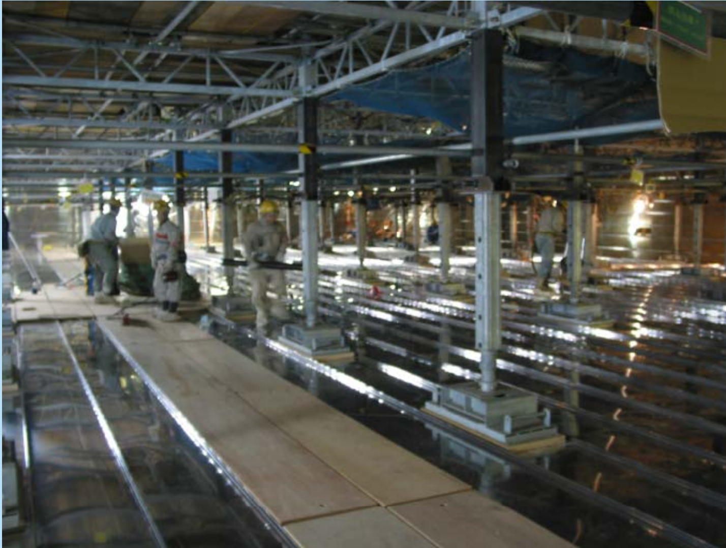
Special staging (12 levels) from bottom to top of a cargo tank for repairs (thousands of pieces of special stage materials similar to the staging in building construction)
